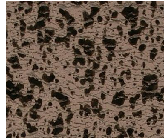
Paint cracking and debonding at a small scale
